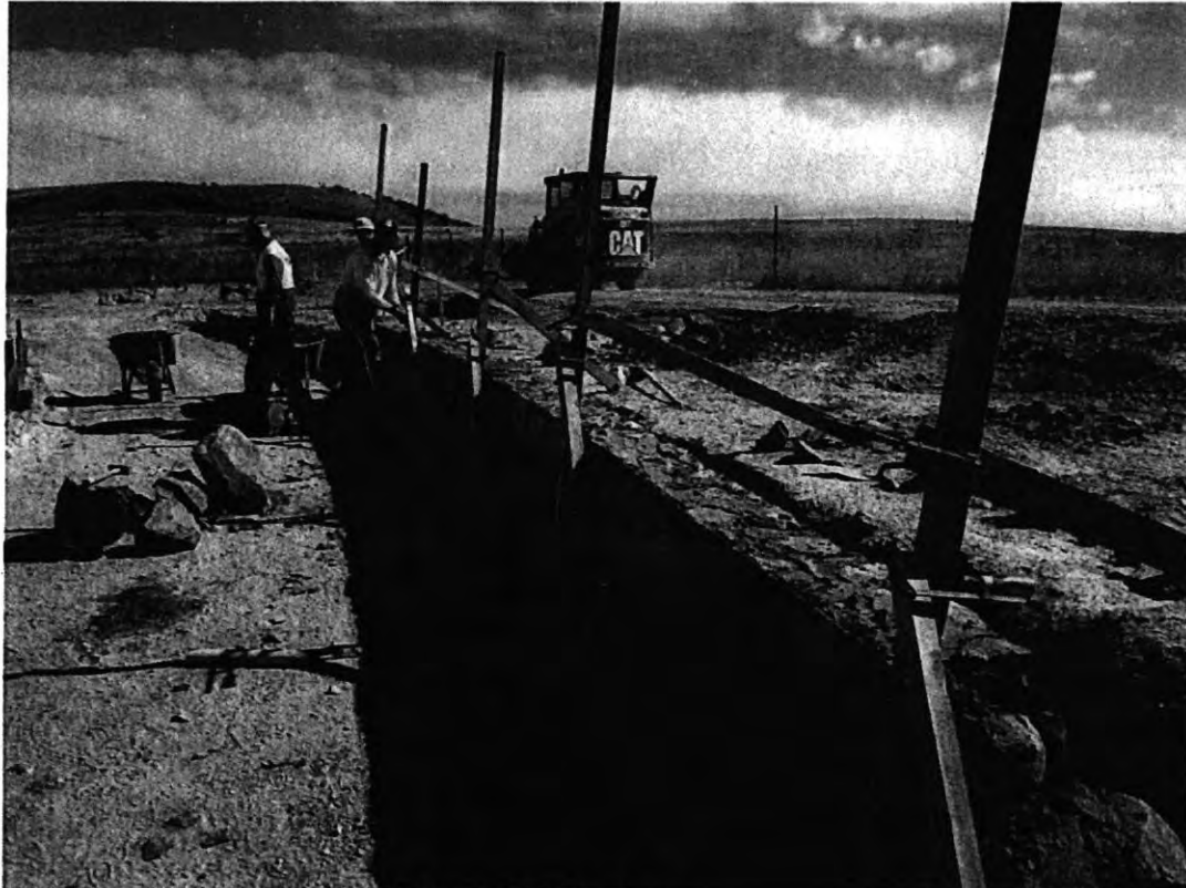
Image 04: Construction of stone pitched retaining wall beside floodway
