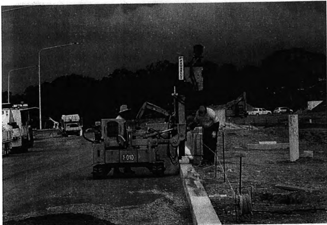
Driving in guard rail posts at CH520
