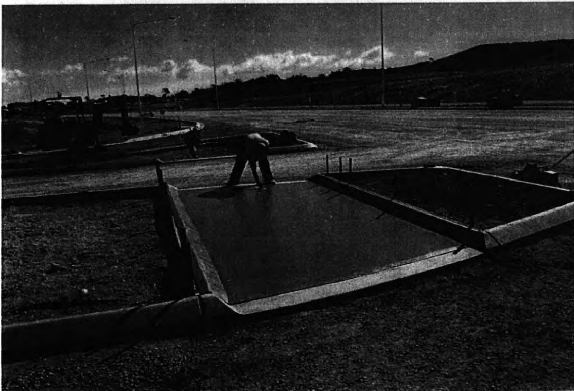
Constructing pram crossing at Road 4 intersection
