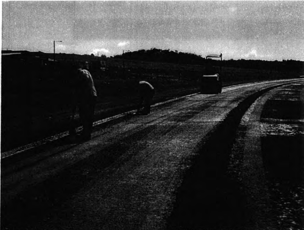
Image 01: Preparation of base material between Burrumarra Ave and the bridge
