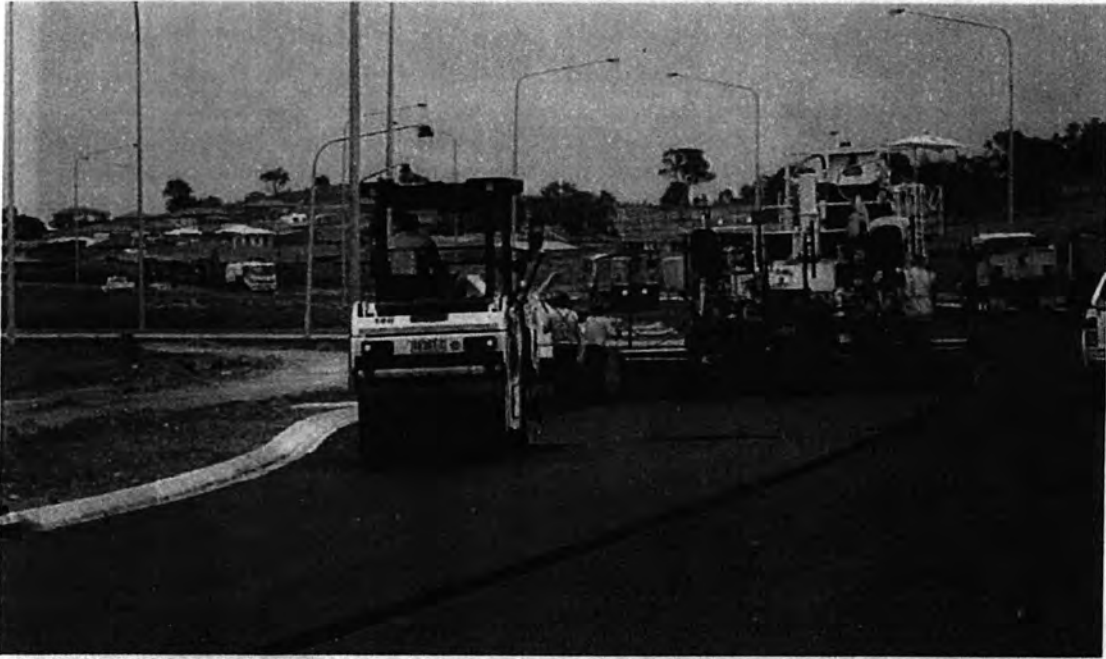
Placement of SMA CH980
