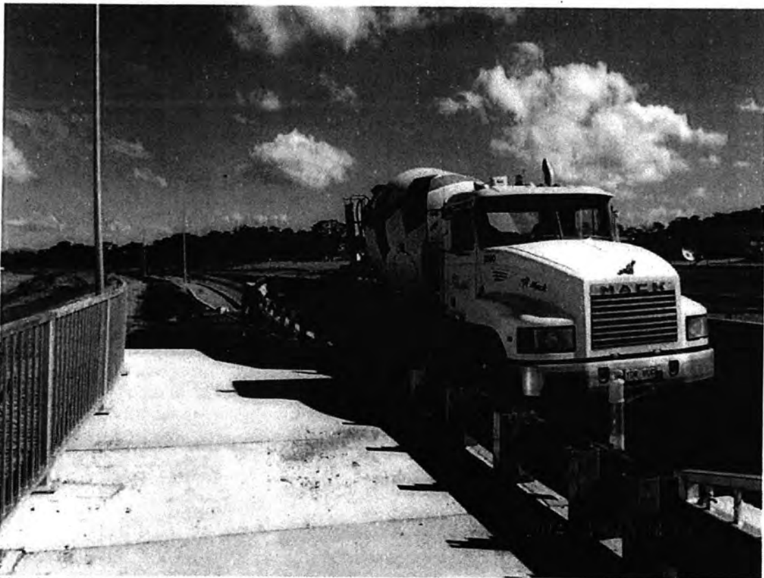
Mowing strips for red granite surrounds being poured
