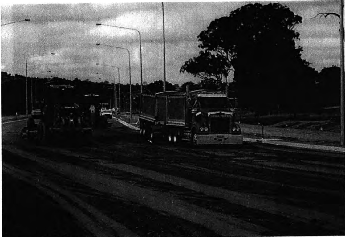
Placement of DGB at CH1000
