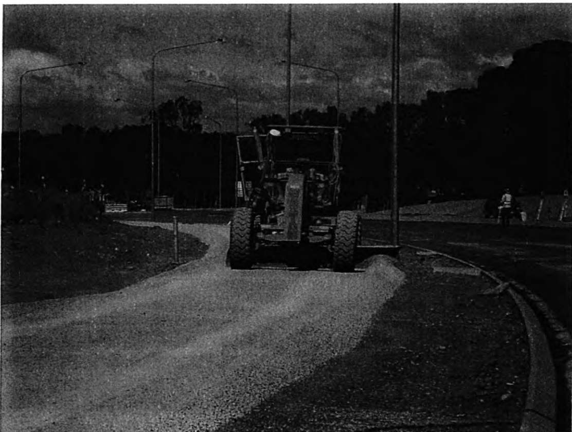
Placement of base for shared path at CH250
