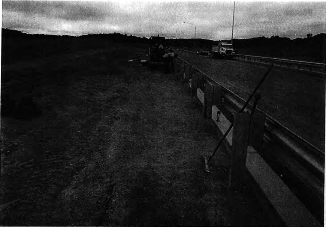
Preparing the base for decomposed granite around the north west guard rail
