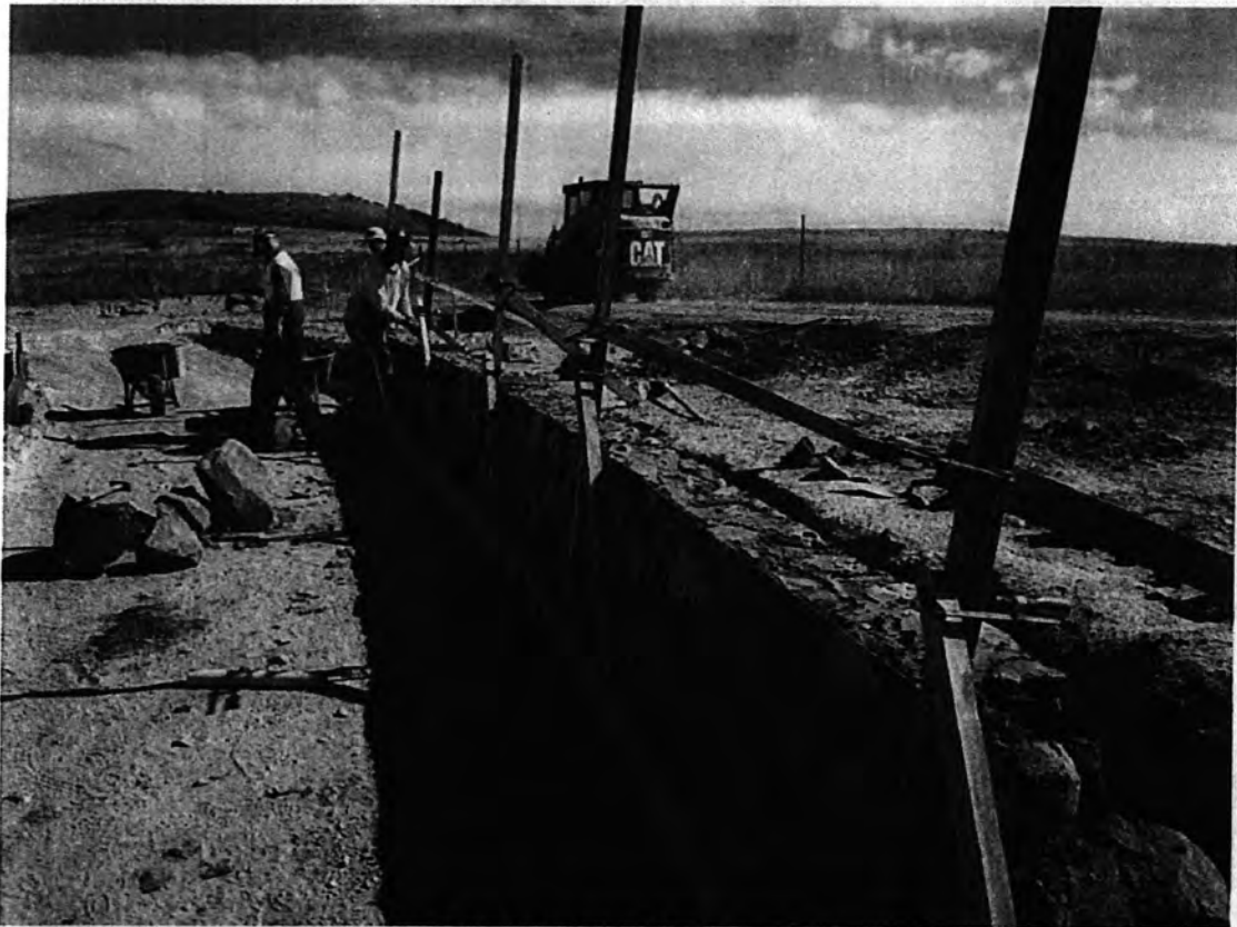
Constructing the equestrian/dhared path retaining wall
