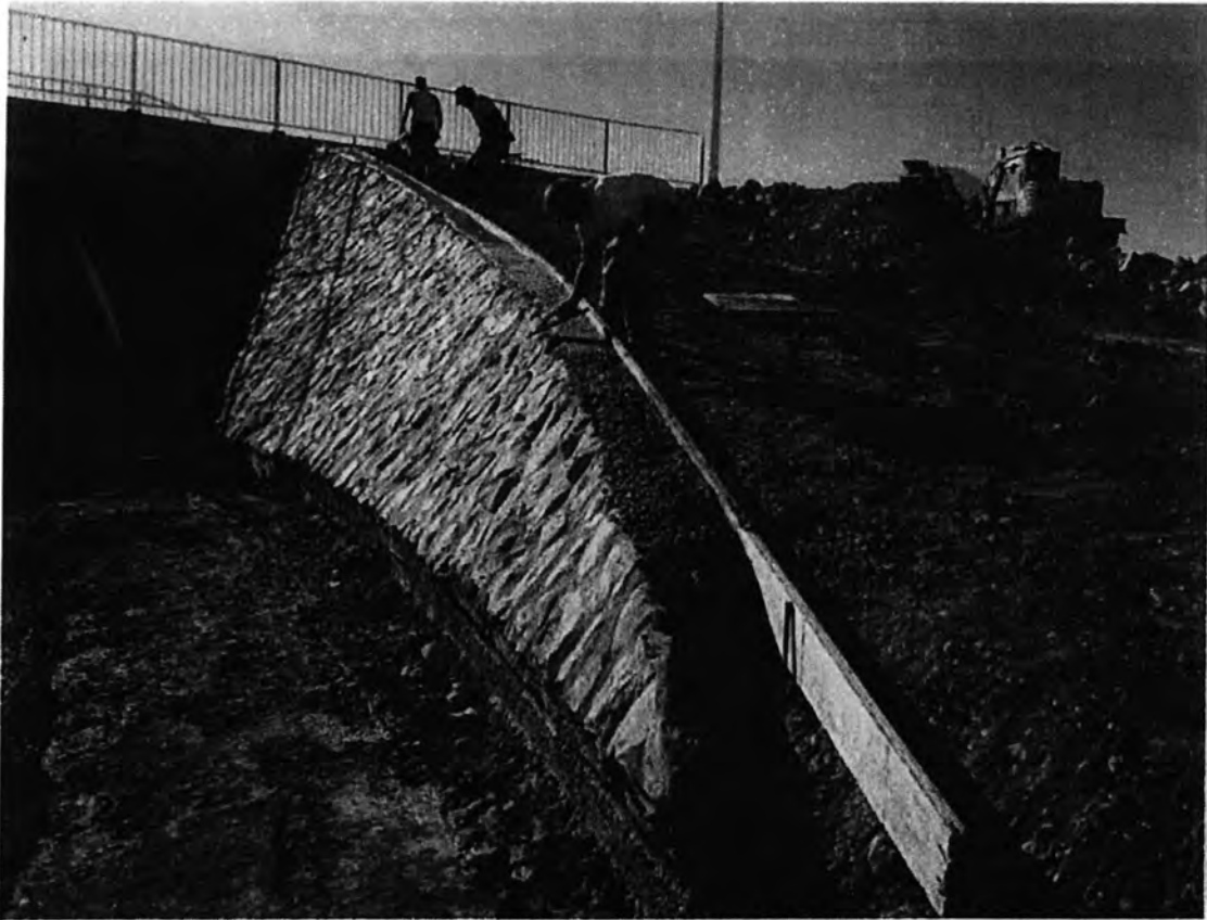
Placement of concrete for north east bridge abutment mowing strip
