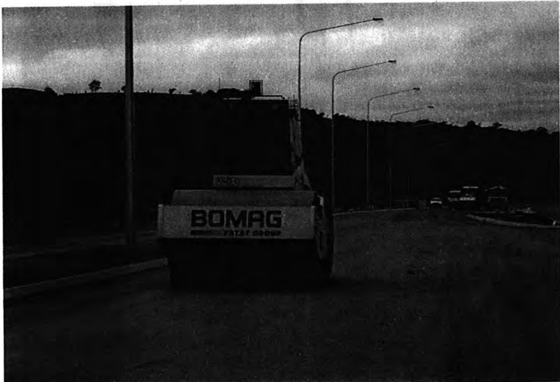
Roller compacting base at CH1080
