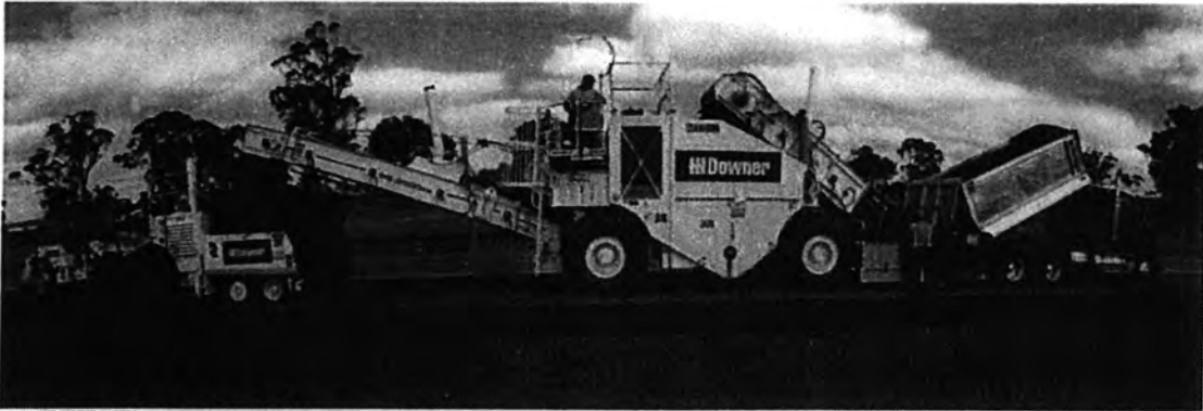
Placement of SMA CH1650
