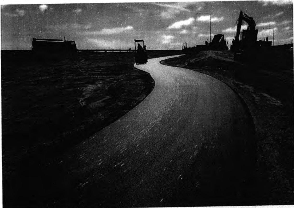
Placement FFG asphalt on the shared path
