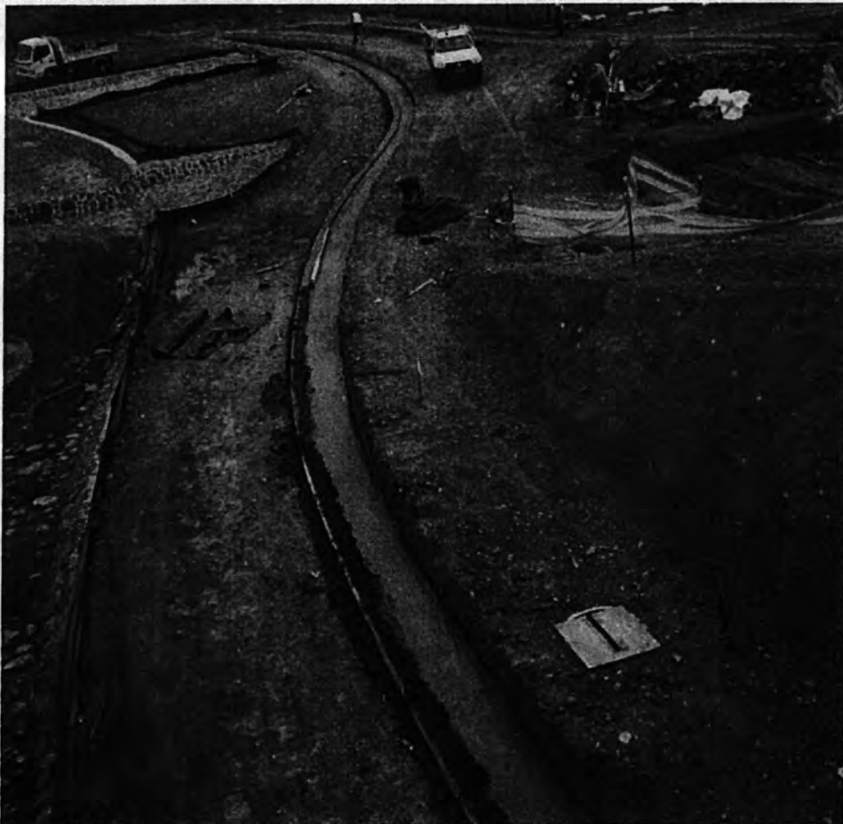
Concrete footing for stone wall at the shared and equestrian path
