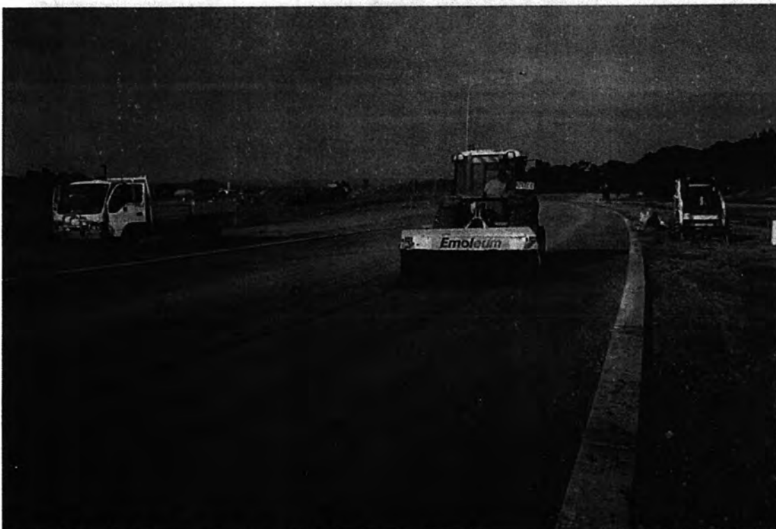
Brooming DGB prior to placement of prime
