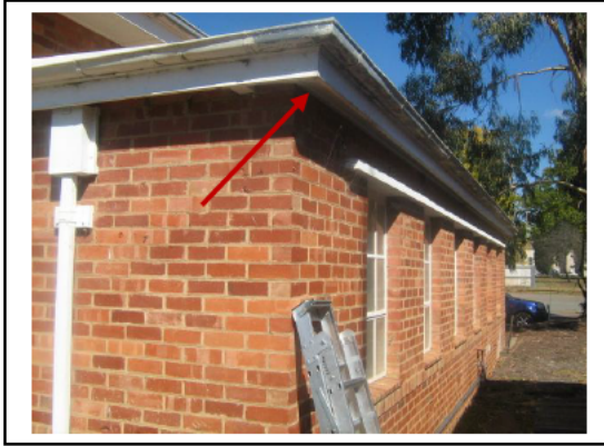
Photograph 1: North west corner of building – eave sheet (refer sample no. 3971 – A7).
