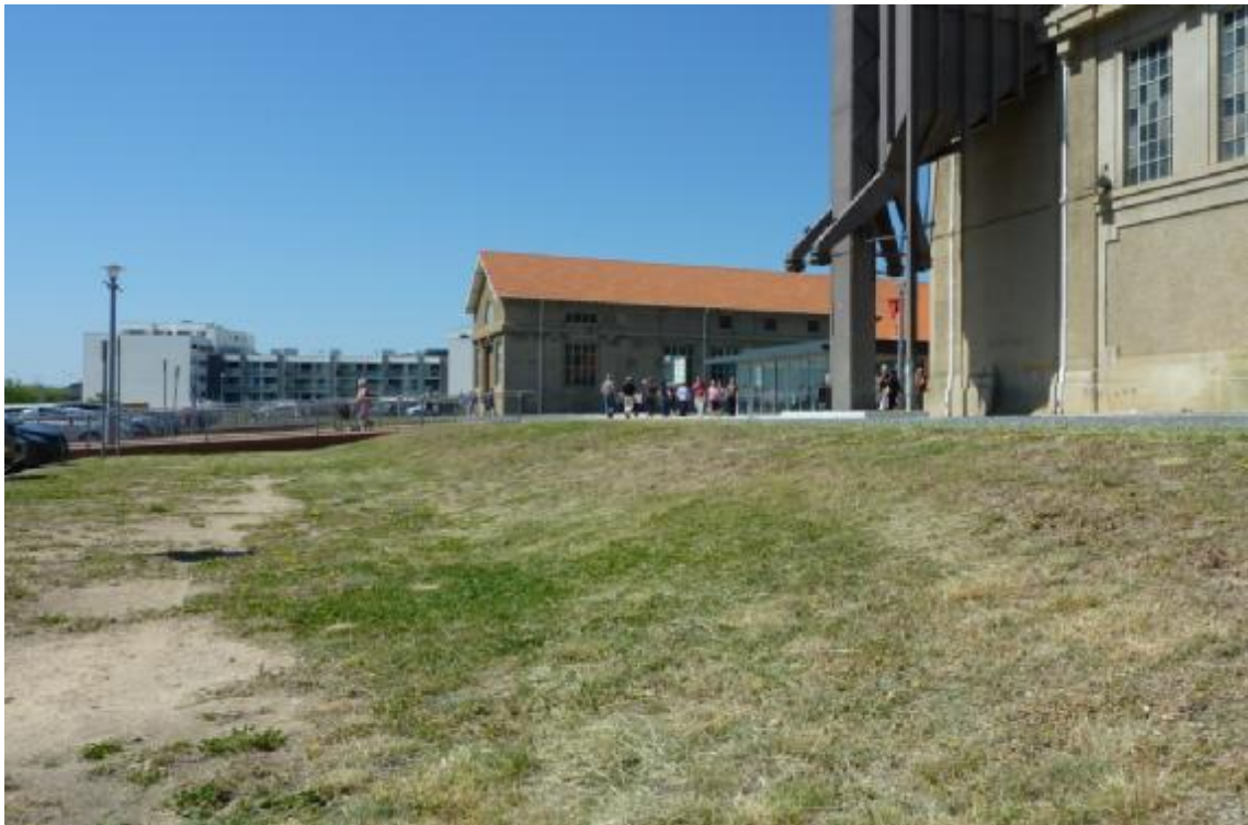
Figure 8 View looking south along the embankment, 2012.
