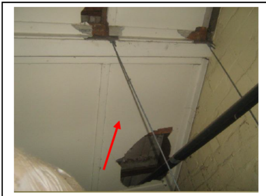
Photograph 3: Main room – ceiling sheet (refer sample no. 3971 – A9).
