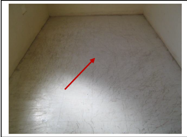
Photograph 4: Store room – vinyl floor tiles (VFT) (refer sample 3971 – A1) No asbestos detected
