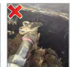
No clearance for Ball valve
