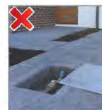
In driveway (unapproved)
